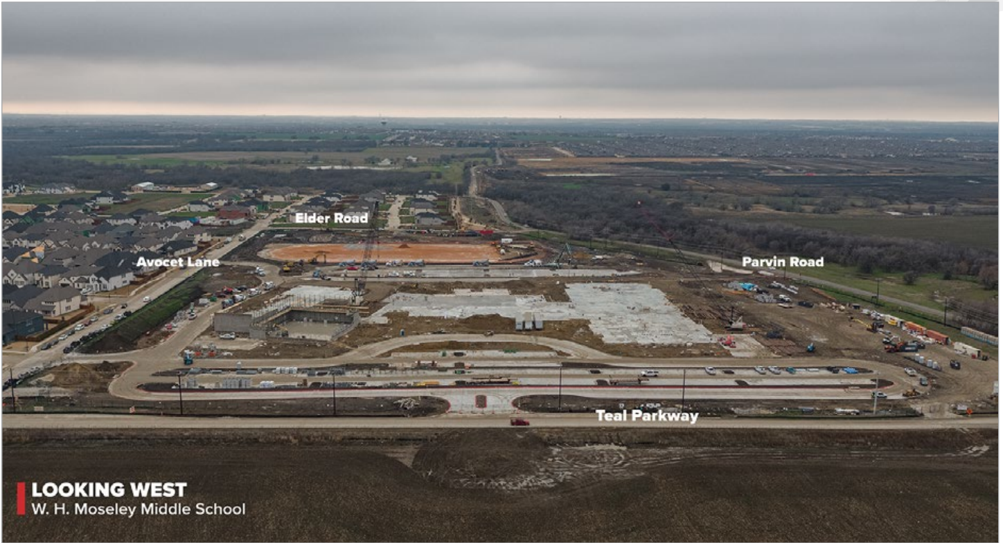
Concrete Drive Placement
