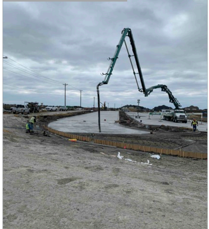
Concrete Site Paving Placement
