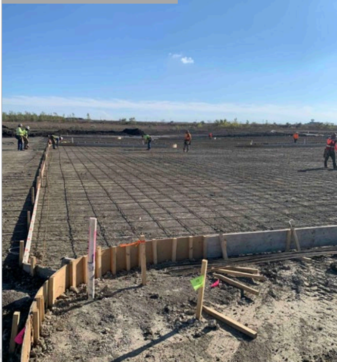
Concrete Site Paving Reinforcing and Formwork
