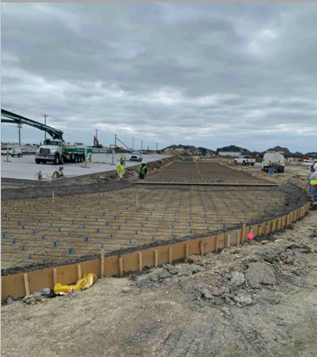
Concrete Site Paving Reinforcing and Curb Placement
