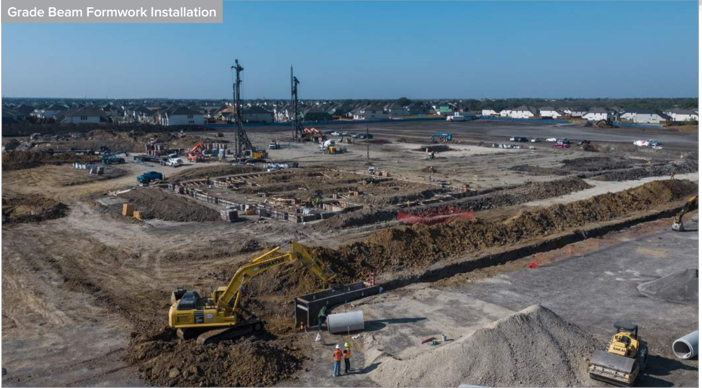
Grade Beam Formwork
