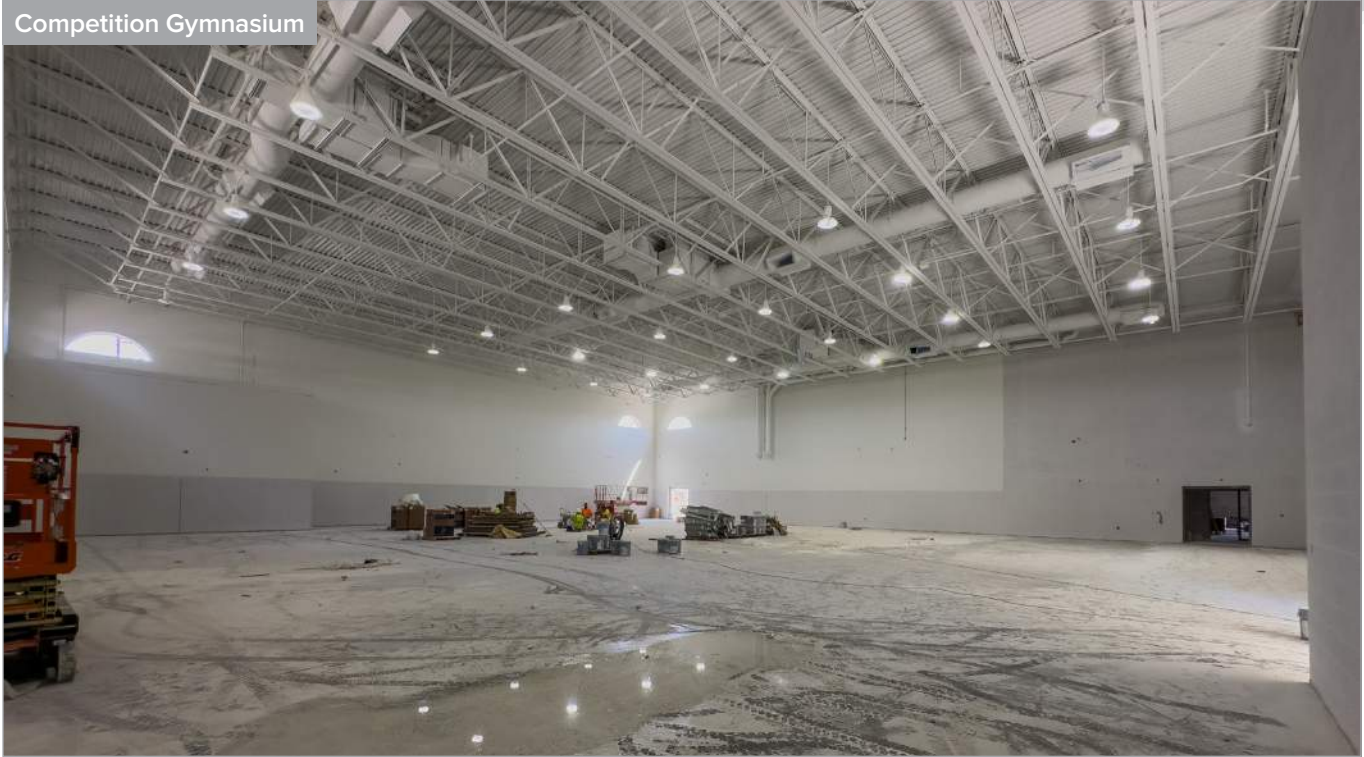
Secondary Gymnasium (Tornado Shelter)
