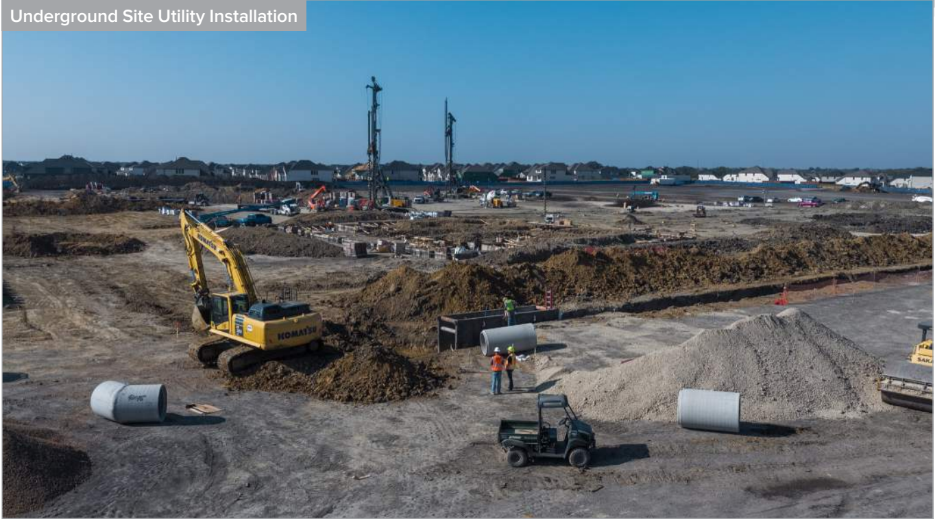
Underground Site Utility Installation
