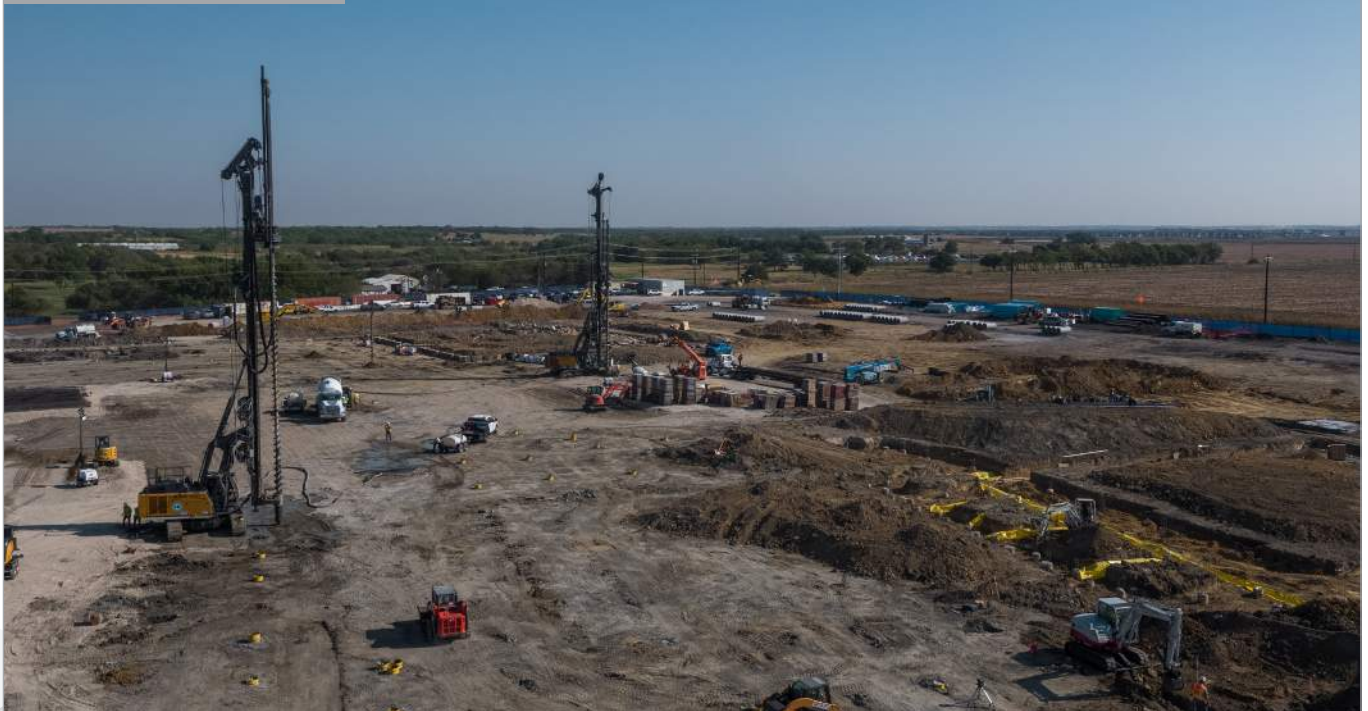
Auger Cast Pile Installation
