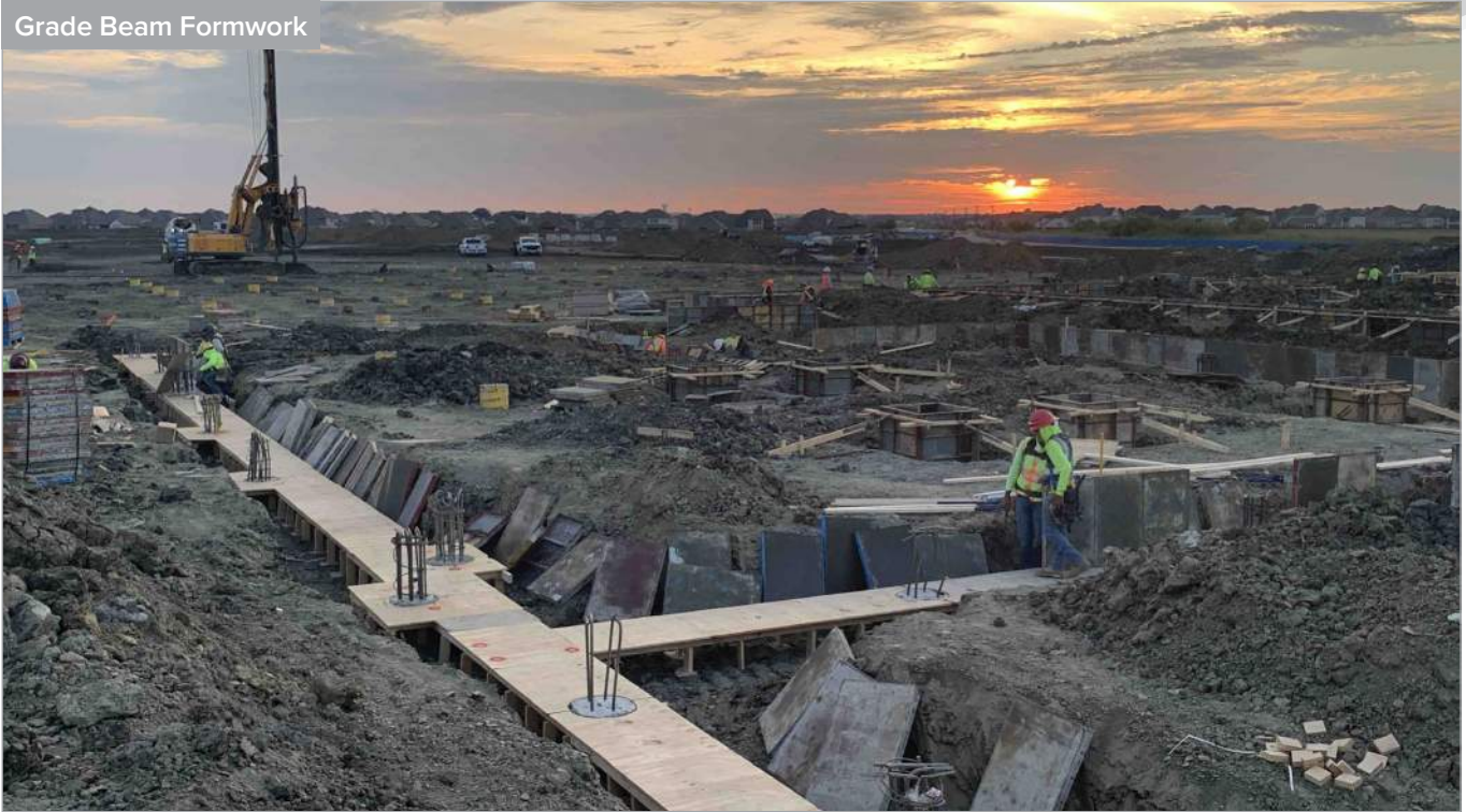
Grade Beam Formwork
