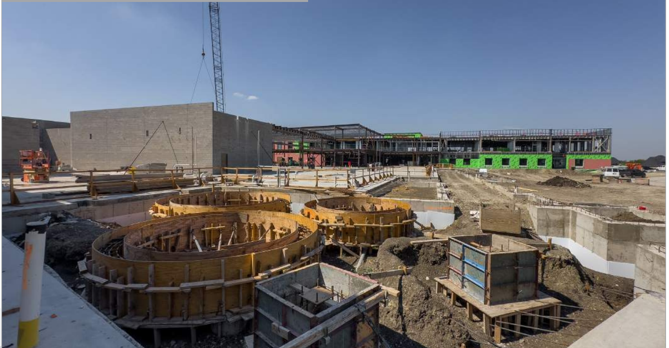
Formwork for landscaped area at Gymnasium Entry
