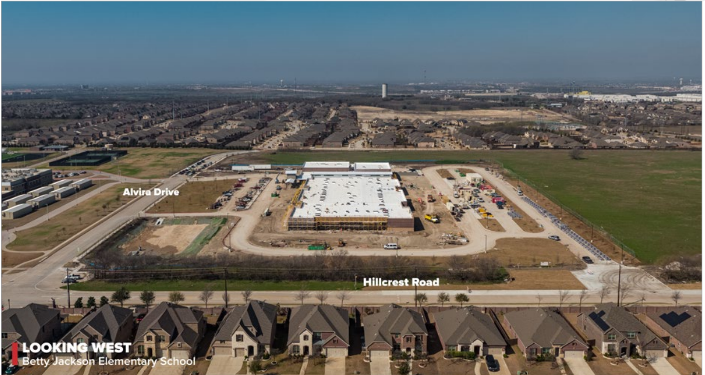
Exterior Masonry Progress
