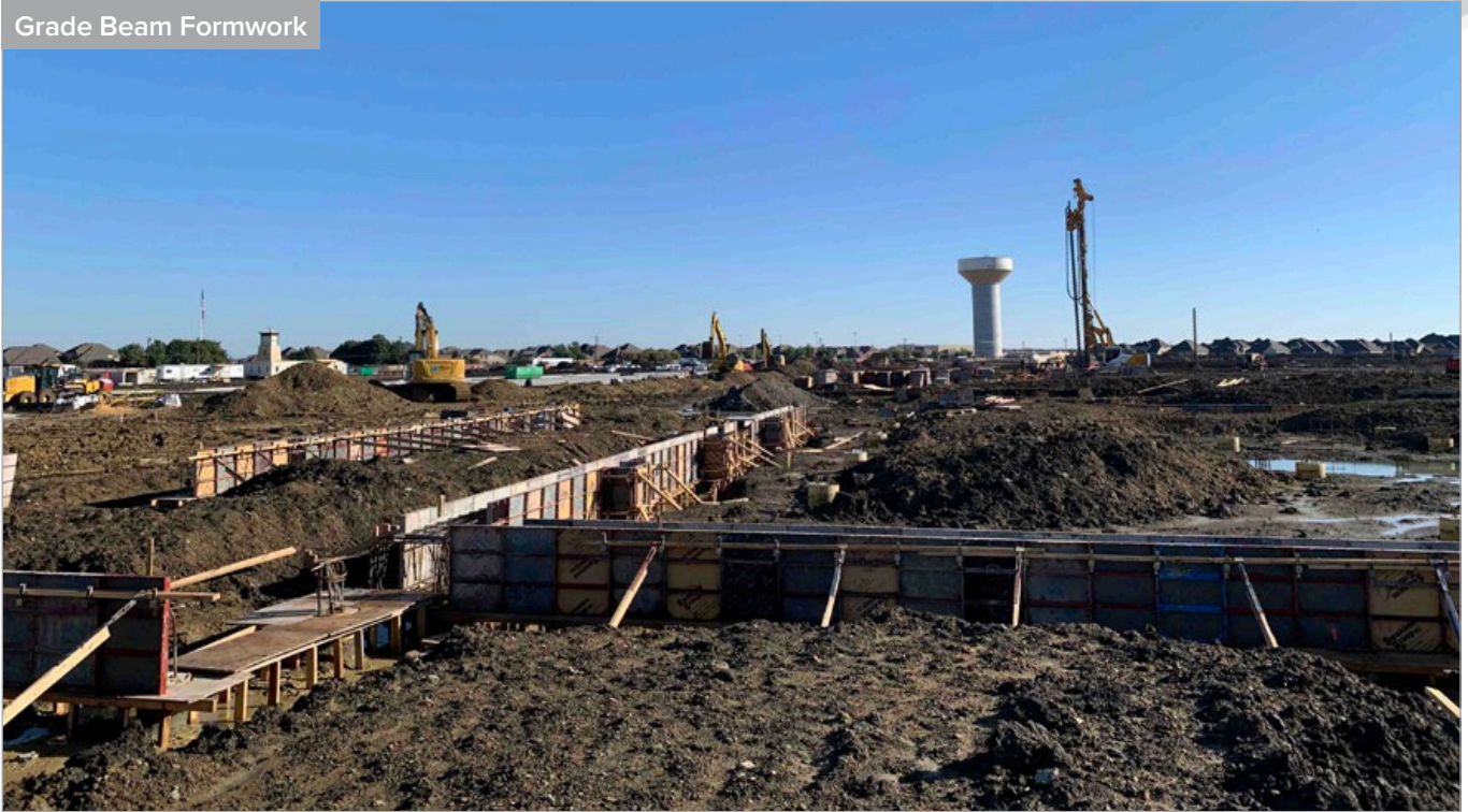
Grade Beam Formwork
