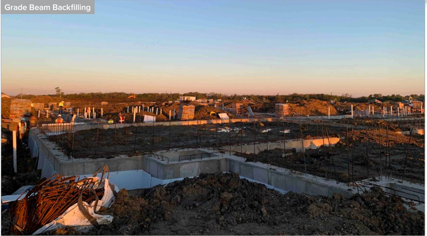
Grade Beam Backfilling
