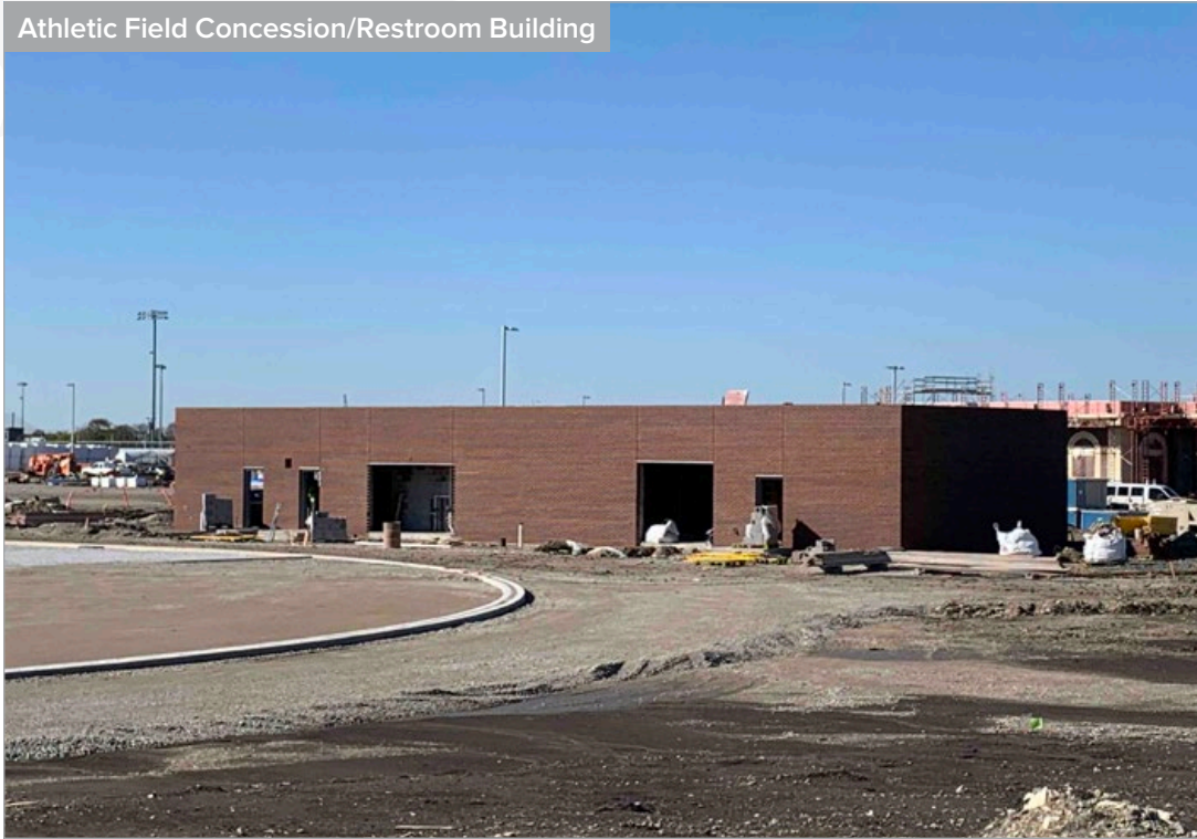
Athletic Field Progress
