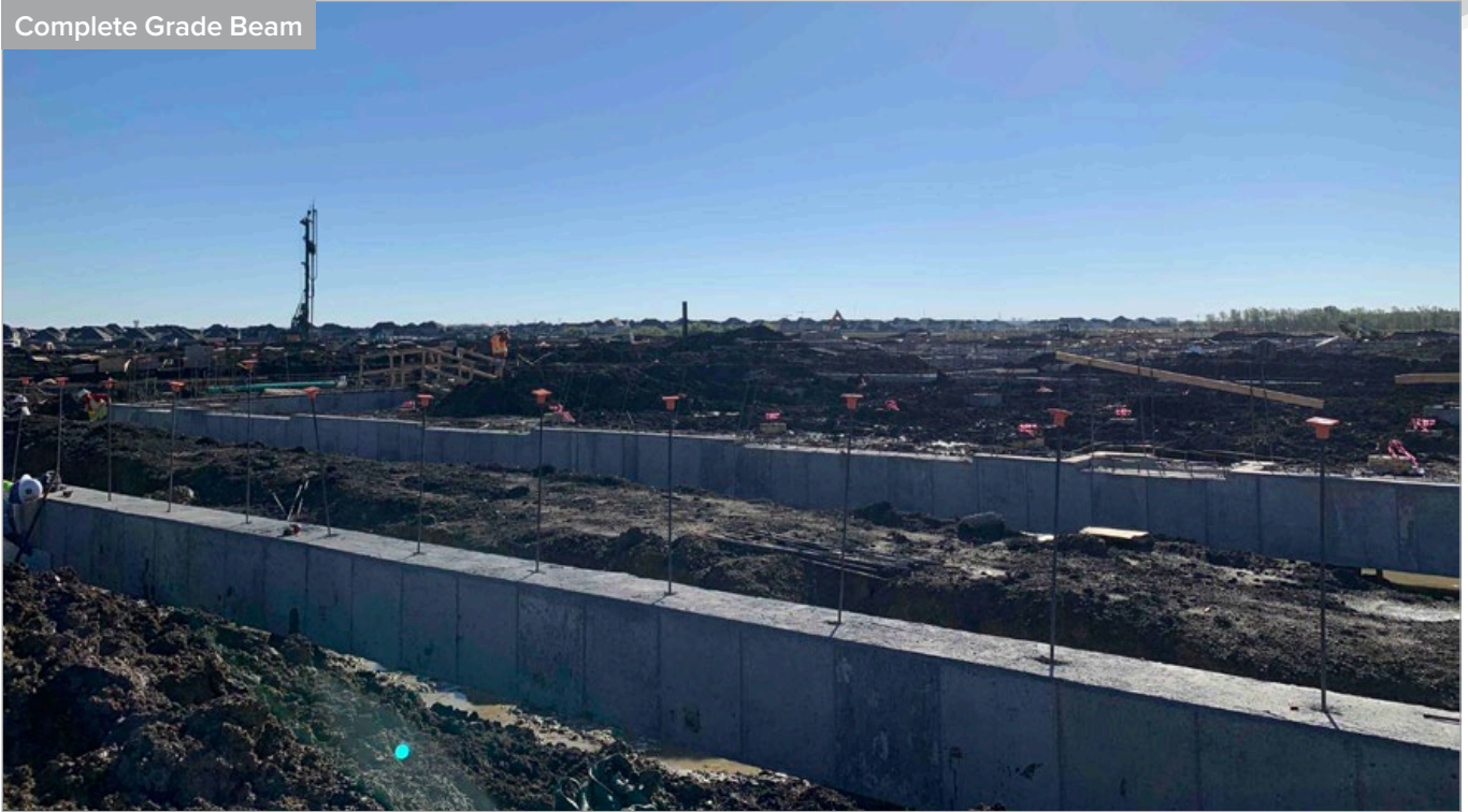
Complete Grade Beam
